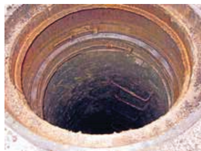
Seal Prior to Removal
