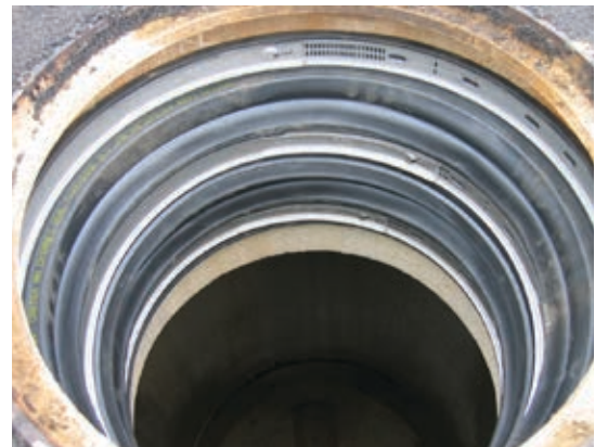
CRETEX INTERNAL SEAL
