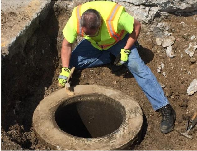
1. Clean the surface of the manhole to be sure no loose material or debris is left behind. Use a chipping hammer or chisel and whisk broom.
