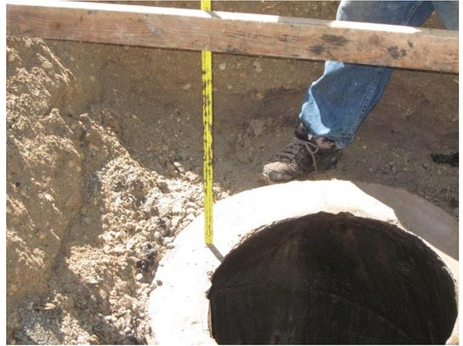
2. Measure the distance from the top of the manhole to the final elevation, subtract the height of the casting and select the rings.
