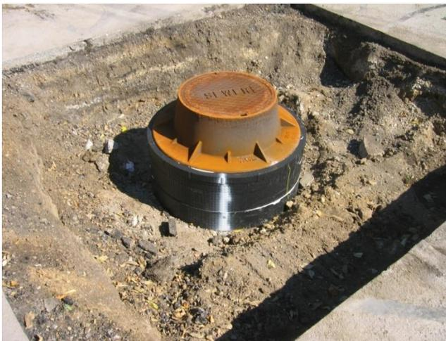
5. If Angle Rings are used, a paint mark should be made on the rings during dry fit to ensure proper position once installed with adhesive.
