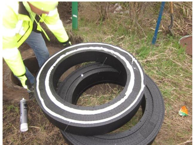
6. Fill both grooves in underside of Grade Ring with M-1 adhesive. Flip the ring with adhesive down onto manhole, making sure it is centered.
