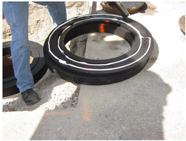
8. Apply M-1 as before to each groove on the underside of the Finish Ring and position with the grooves down onto the Grade Ring.
