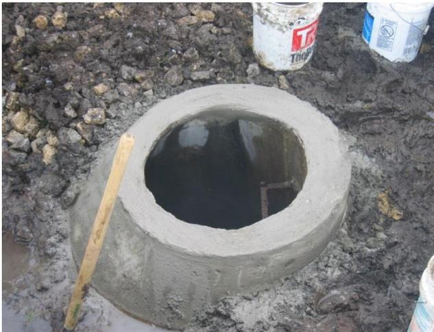
3. If necessary, repair any manhole surface defects with a non-shrink repair mortar to ensure a level surface and prevent point loading.
