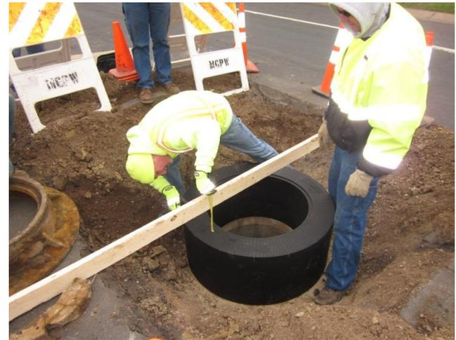
4. Dry stack the selected rings and verify the measurements to ensure the desired elevation has been attained.
