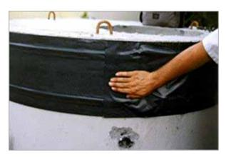
3. Remove protective film from the closing flap to cover the two tensioning ratchets and straps, completing joint. Cretex Wrap equipped with high tensioning ratchets provides a positive seal on box, arch, elliptical and round pipe.
