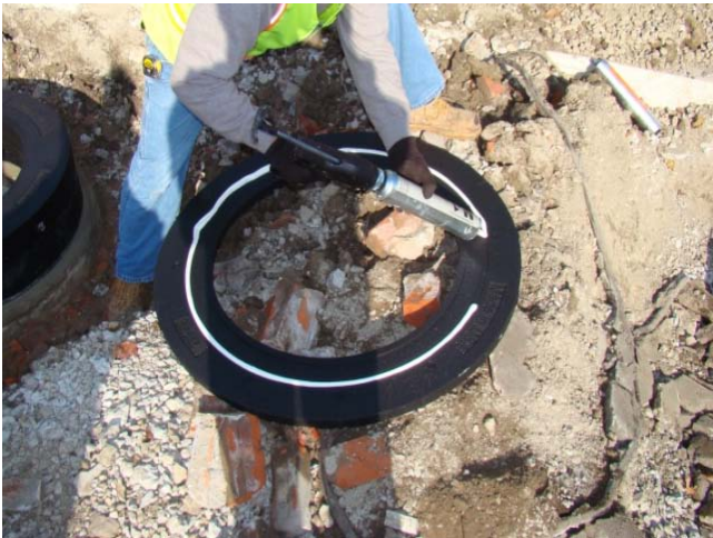
9. For Angle Rings, place a ¼” bead of M-1 into the groove on the underside of the Angle Ring and to the inside shoulder of the Finish Ring.
