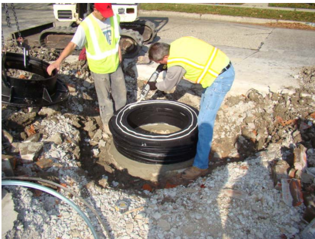
11. Place two ½” beads of M-1 adhesive on the top surface of the Finish or Angle Ring prior to setting the manhole frame casting.
