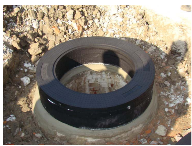
8. Apply M-1 as before to each of the tongues and position the Finish Ring with the grooves down onto the Grade Ring.
